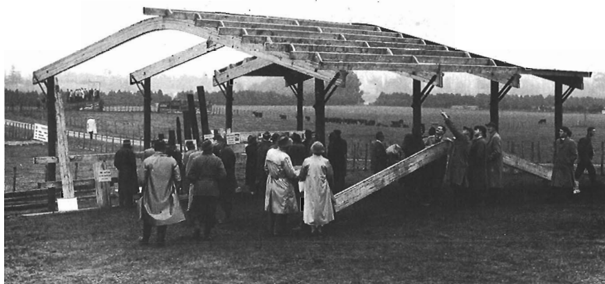
A Forest Service exhibition of material available to the farmer, including the laminated truss barn, at a Farmers' Day at Ruakura Animal Research Station in June 1961.
