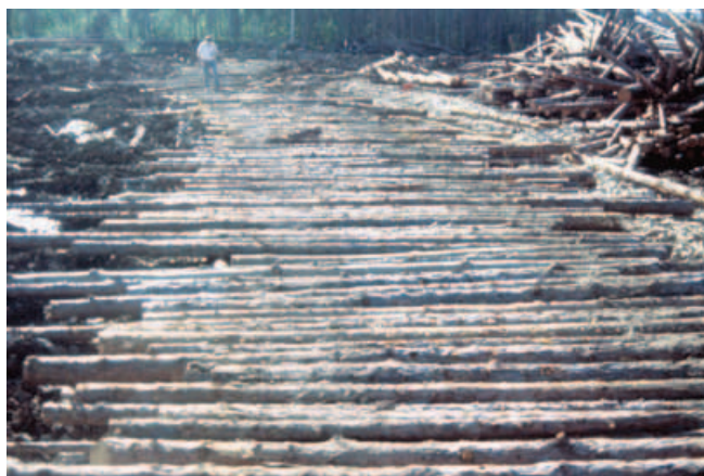
A corduroy of small logs for log extraction
