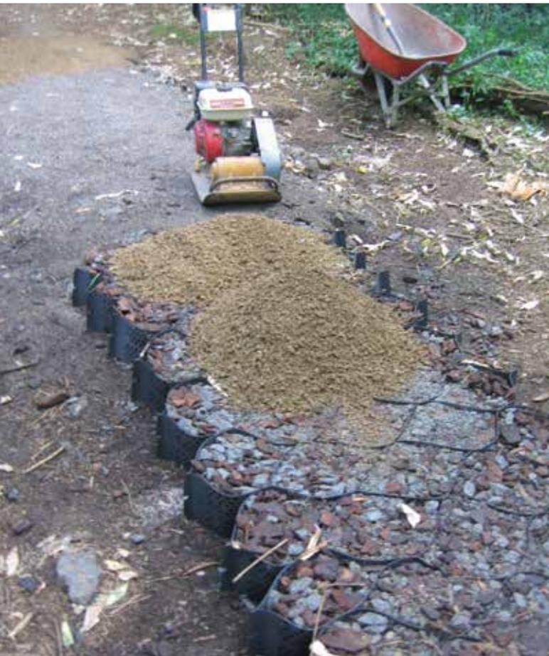
Installing geoweb on a DOC track in 2009 to trial the geoweb system
