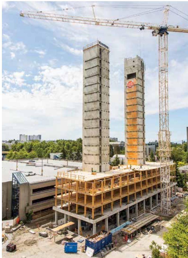
The use of CLT panels for the stair and elevator cores was considered for the project, but concrete helped streamline the structural design (in particular the lateral resistance) and reduce costs, as well as simplify the already complicated permitting and approval process. Photo courtesy of naturally:wood
